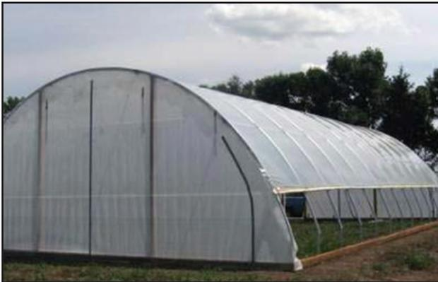
The frames, which can be constructed of metal pipe, wood, or PVC pipe, are covered with one or two layers of greenhouse-grade polyethylene; those covered with two layers of plastic have an air layer in between, thus offering better insulation and, consequently, more cold protection.
